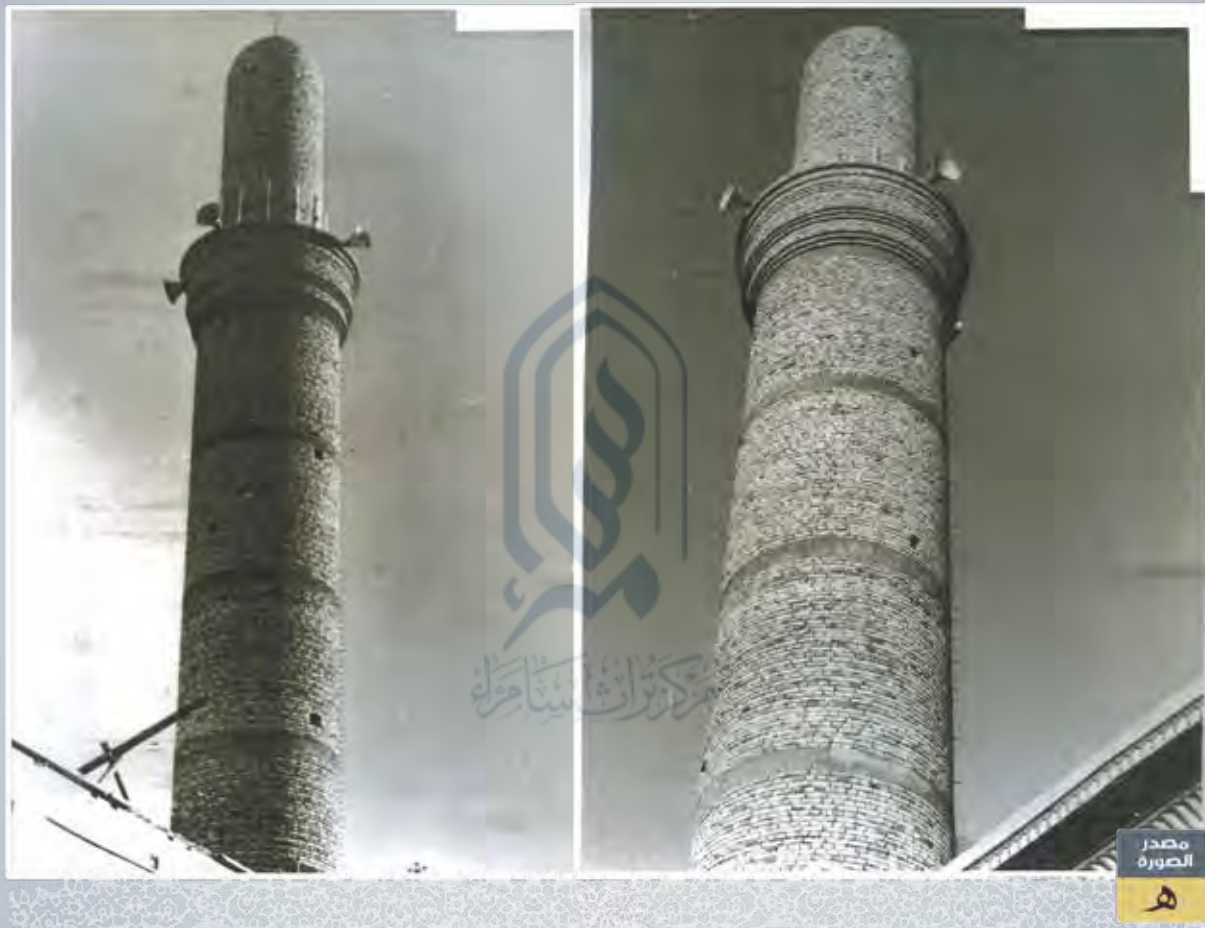
1978 A.C: Holy Al-Askari Shrine Minaret before Renovating.
