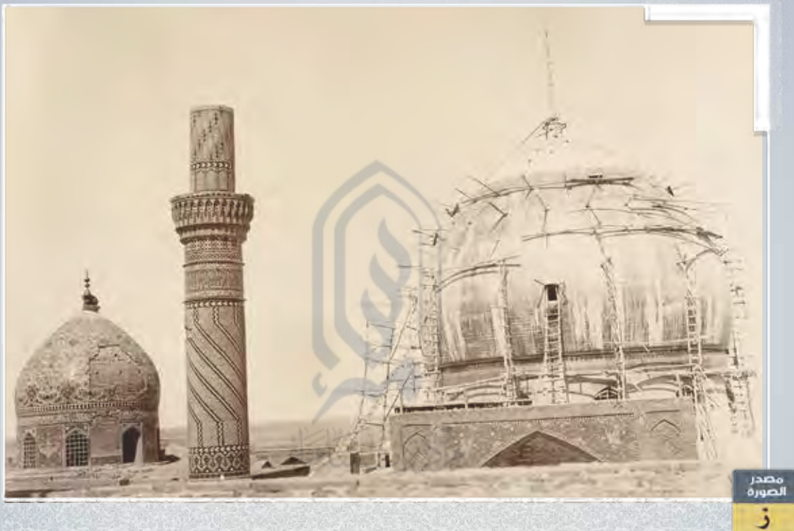
Samarra 1905 A.C: Renovation and Rehabilitation of the Two Holy Al-Askari Imams Shrines Dome.
