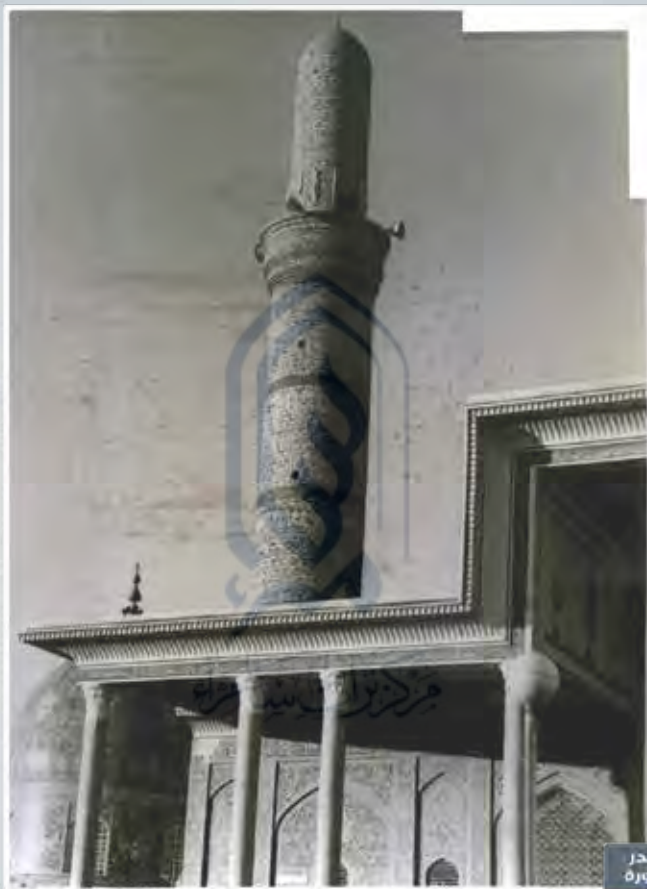
1978 A.C: Holy Al-Askari Shrine Minaret before Renovating.
